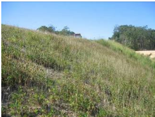
Photo 1. In January 07 Fill batter 6B shows a good progress with surface coverage of perennial grass cover. There is also evidence of native vegetation germinating.
