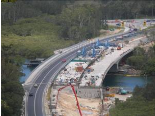
Photo 13: Brunswick River Bridge work site during February 2007.
