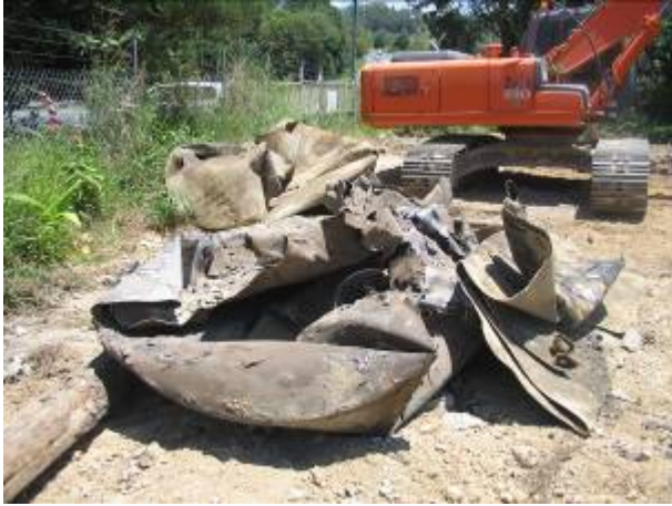
Photo 15 and 16: Disused underground storage tanks exposed, and removed from site.
