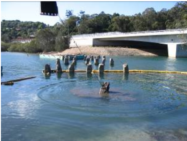
Photo 10: Old bridge pile being removed.
