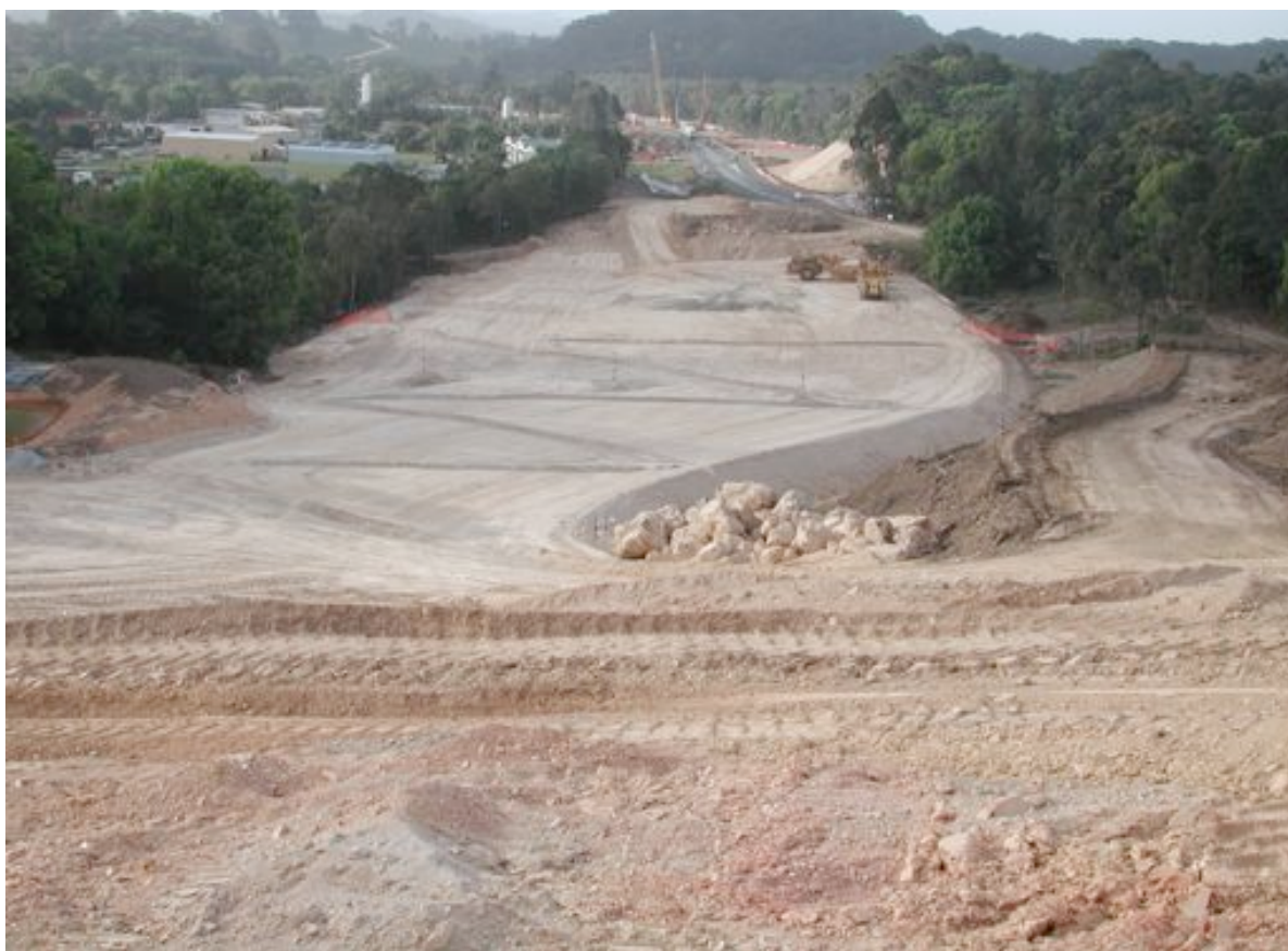
Photograph 3.3 Major earthworks being undertaken close-to Billinudgel with associated high dust risk.
